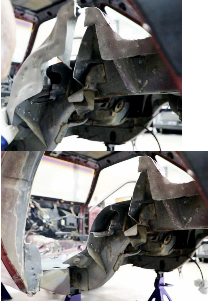
Figure 19 - Remove Front Factory Structure
