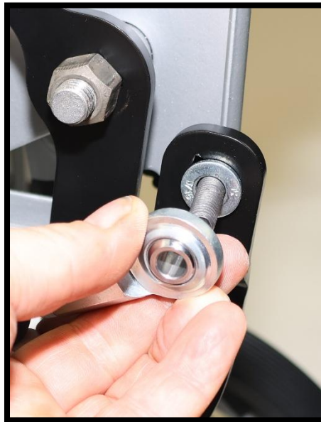
Rod-end being installed
