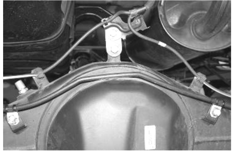
re-install A.B.S. line back into plastic clips
