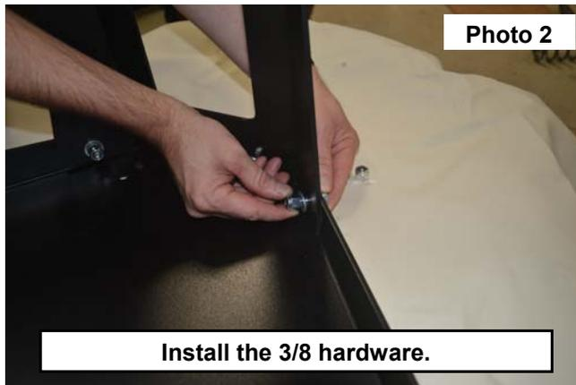
2. Torque the 3/8 hardware to 35 ft-lbs. using a 9/16 wrench and socket. **See Photo 3.**
