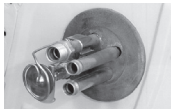
Photo 10 - Install Round Grommet
