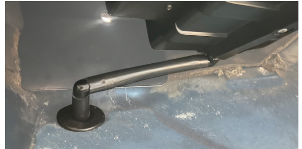
Photo 12 - Install Drain Tube
