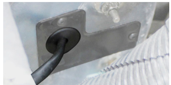
Photo 23 - Route Heater Valve Wire Harness through Block-off plate & grommet
