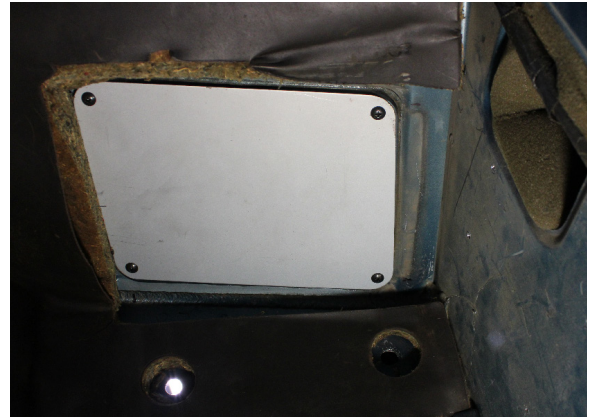
Photo 3 - Install Fresh Air Block-off plate.
