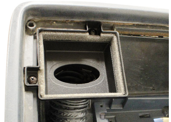
Photo 16 - Install Driver Side Duct Adapter
