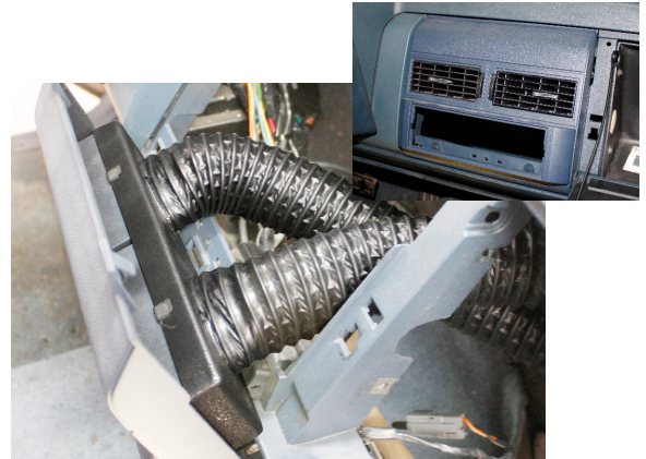
Photo 27 - Install Duct Hose & Center Vent
